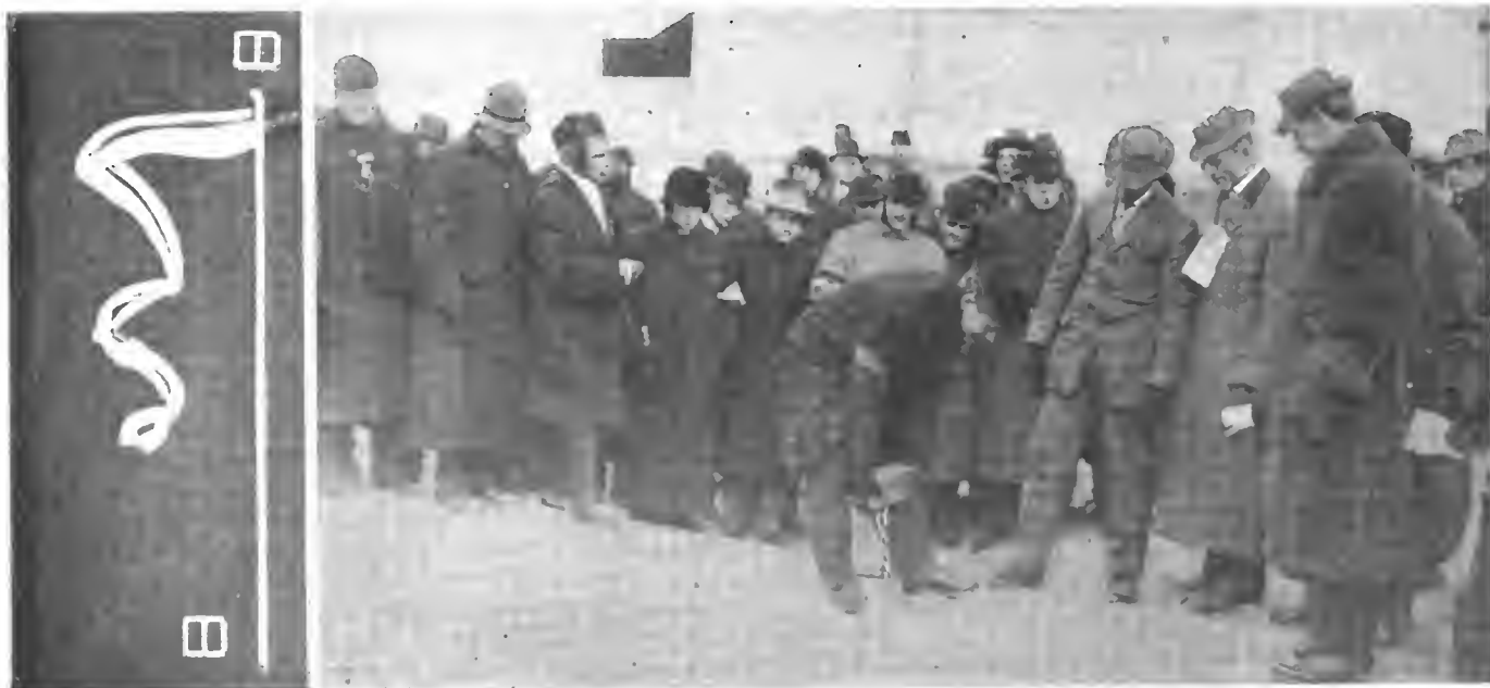
Governor Marshall, of Indiana, Placing the Golden Paver Which Completed the Track into its Position
